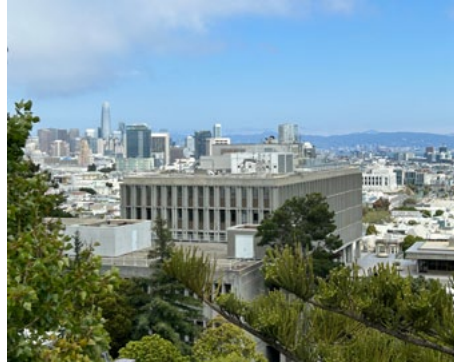
Exposed HVAC equipment on CPMC's roof is evident in this view of the campus from above Castro Street.
