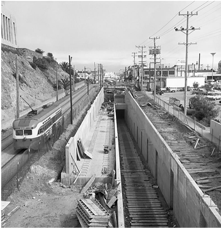
Figure 102. Construction of the entrance to the Muni Metro tunnel at Church Street and Duboce Avenue, 1972. Source: SFMTA Archives, Image No. M1273_3
